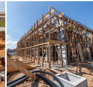
UBS Maringá: 38,28% executada
